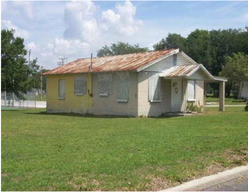
Dilapidated single-family structure
