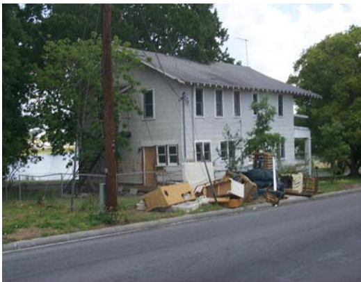
Blighted multi-family structure
