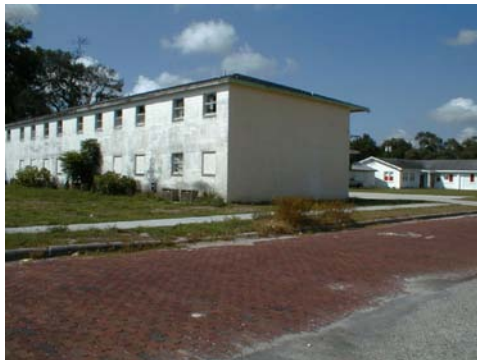
Dilapidated apartment building
