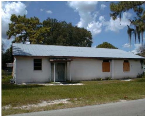
Unsafe single-family residence
