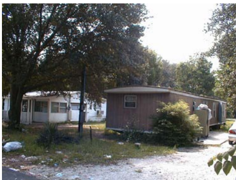
Unkempt mobile home park
