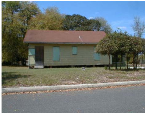
Boarded-up single-family residence
