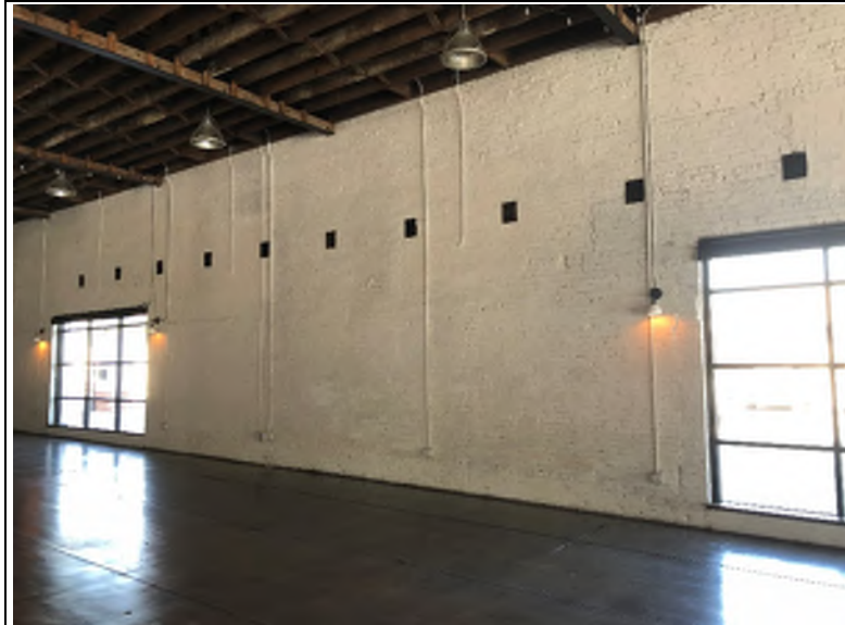
Photo No. 3 Interior view of Test Area #1, and #2
